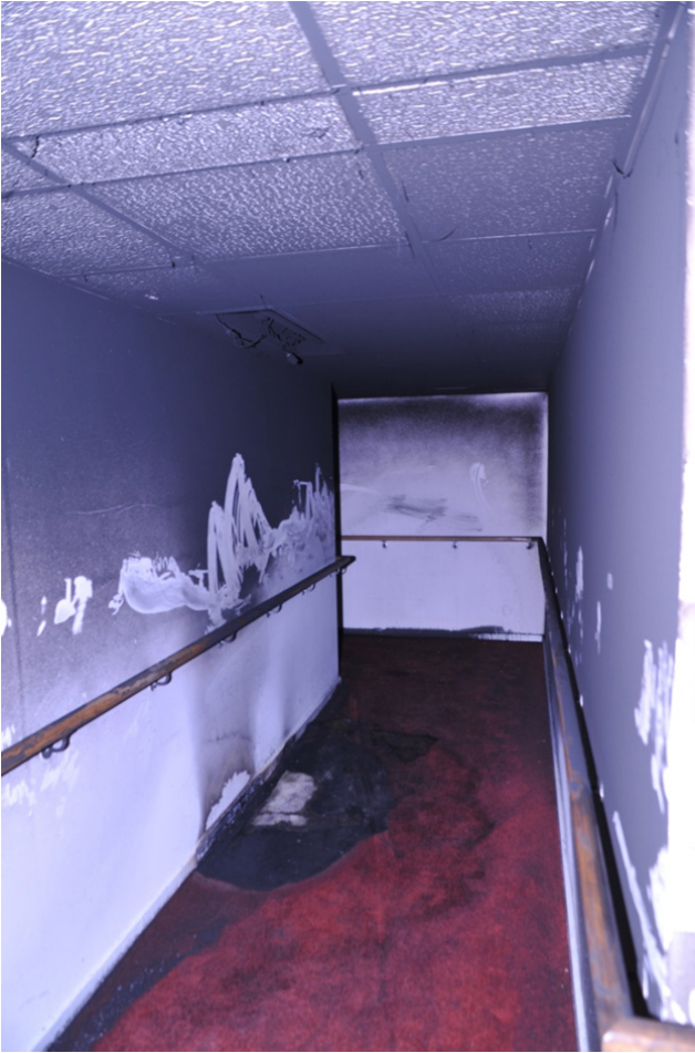
Photo 3 – Seat of fire and light fitting above
