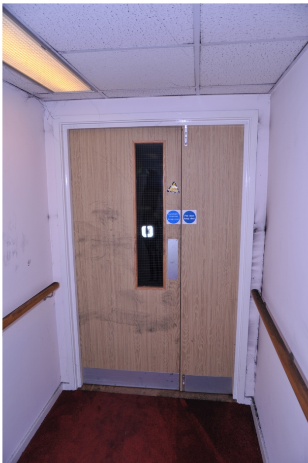
Photo 1 – Corridor immediately outside the fire compartment
