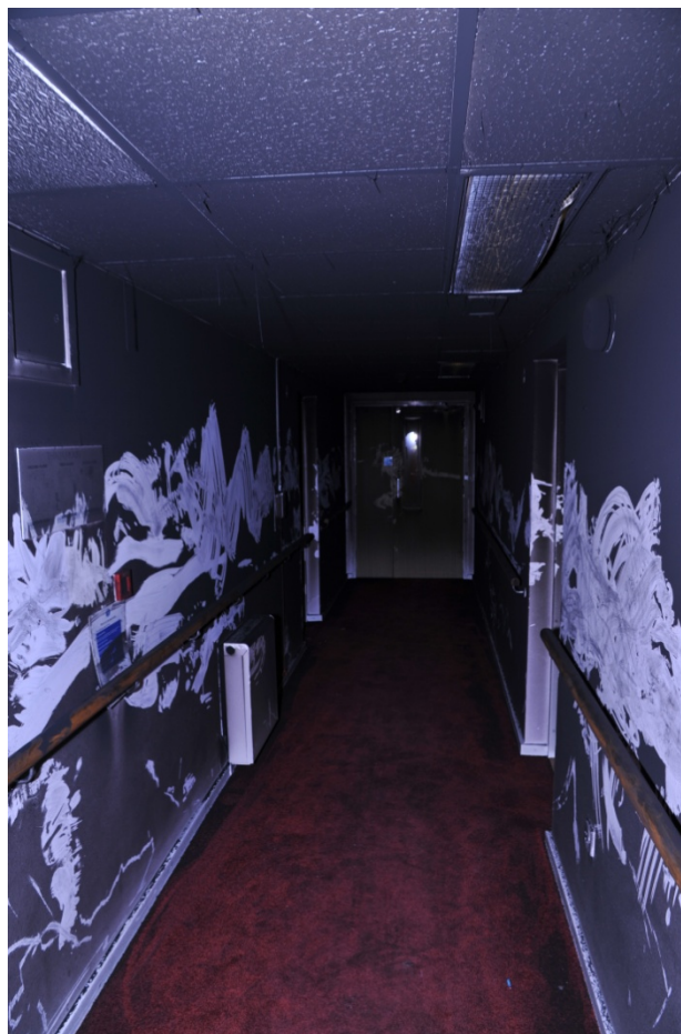
Photo 2 – Inside the fire compartment
